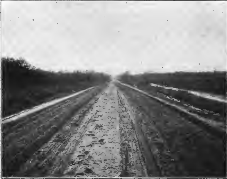
CORLISS AVENUE, OCEAN GROVE, MONMOUTH COUNTY, BEFORE IMPROVEMENT.
